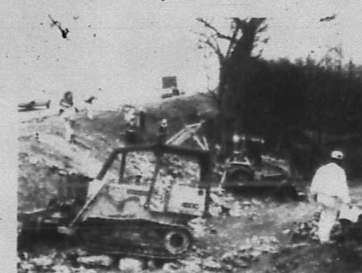
Armando Martinez of Houston watches his Pipeline Construction Co. crew as they prepare a section of State Highway 16 to receive concrete rip-rap. The road construction is part of the continuing repair work being done to undo the damage caused by back-to-back flooding in May and June.
