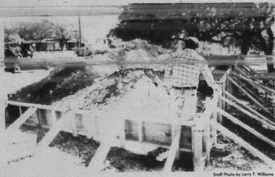
Contractors prepare the foundation formwork for the new Mission Bautista, now under construction near the First Baptist Church in Bandera.
