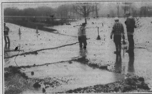
Probably the most damage in the county occurred when the approach to the Tarpley Bridge (FM Road 470) washed out. Workmen here survey the damage.
